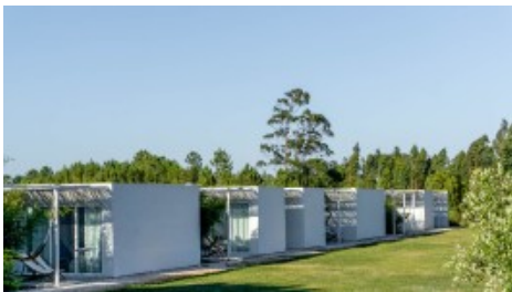
Exterior Area and Playground
