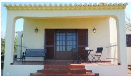
Casa A - south terrace
