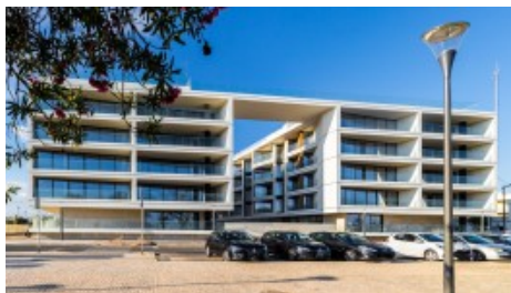
Front of property
