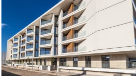
Side of property
