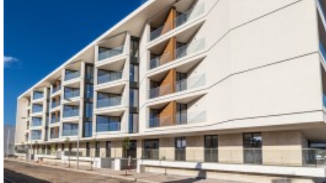
Side of property
