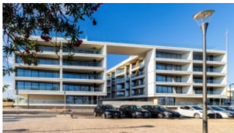
Front of property
