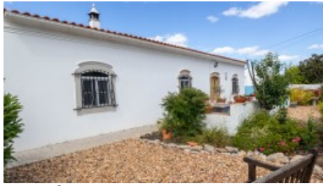
Front of property
